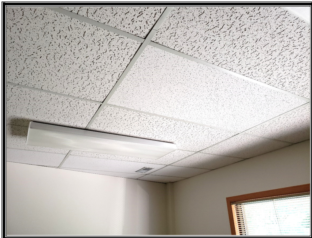
Photo 10: Viewing at two styles of acoustical ceiling panels in the Marshall Financial Group unit.
