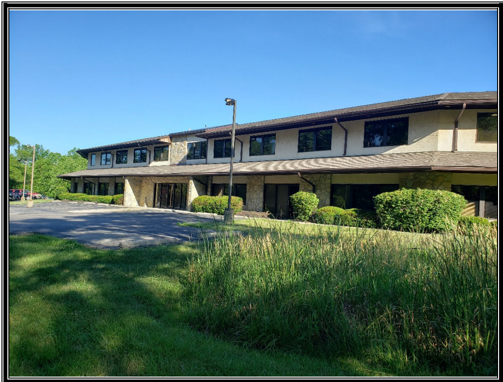
Photo 4: Viewing at the south side of the office building.
