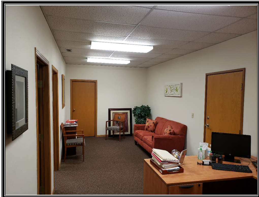
Photo 9: Viewing at the lobby in the Marshall Financial Group unit with acoustical ceiling panels, drywall, and carpet..
