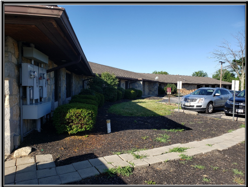
Photo 2: Viewing at the north exterior of the office building.
