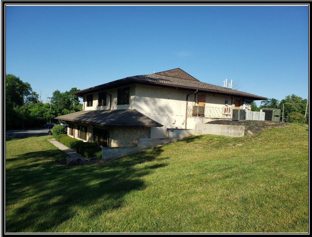
Photo 3: Viewing at the east side of the office building.
