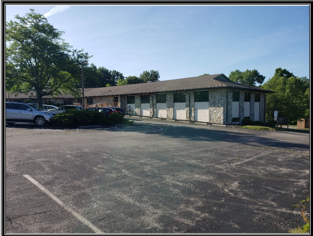
Photo 1: Viewing at the northwest exterior of the office building at 1418 Brice Rd.
