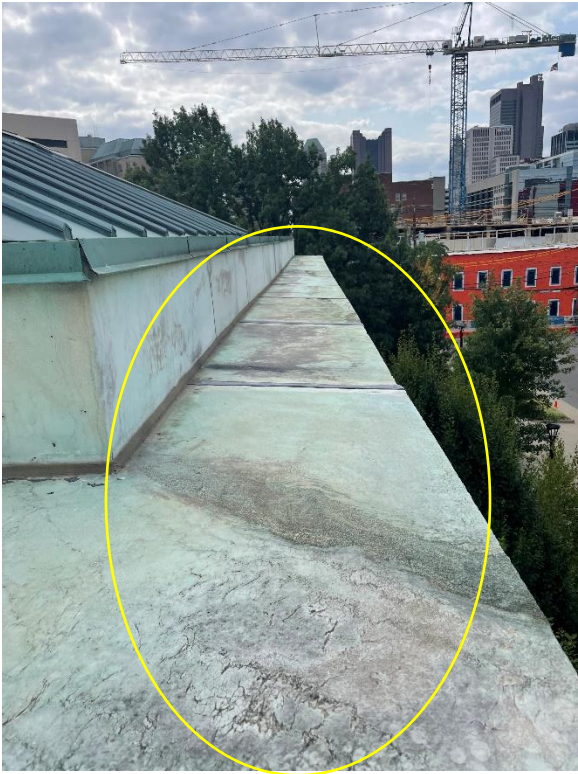
South facing top side of horizontal cornice capstone ledges
