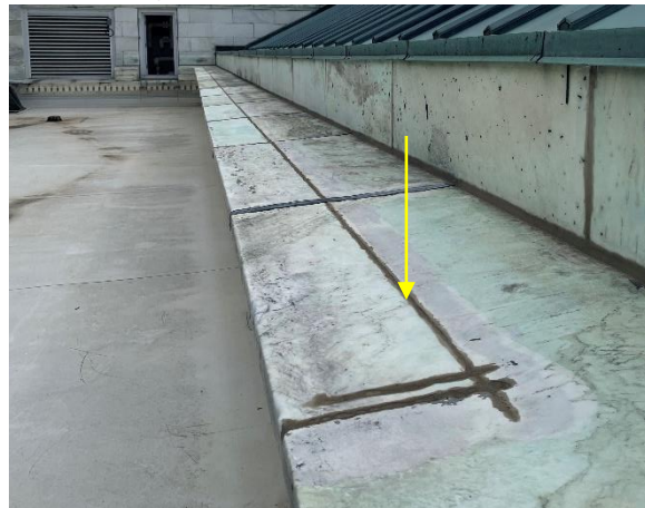
Horizontal joints on cornice stones
