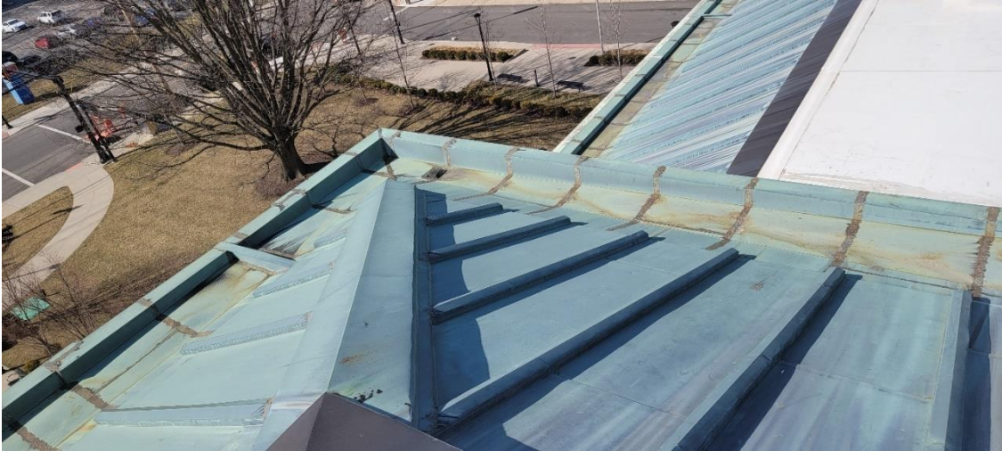
Integral Box Gutter center portion northwest corner
