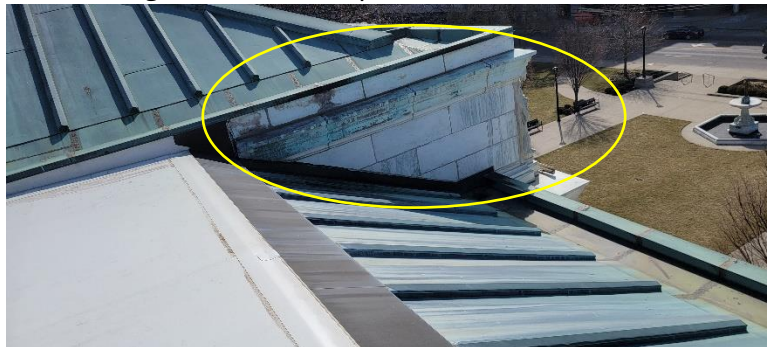
North facing vertical marble panels
